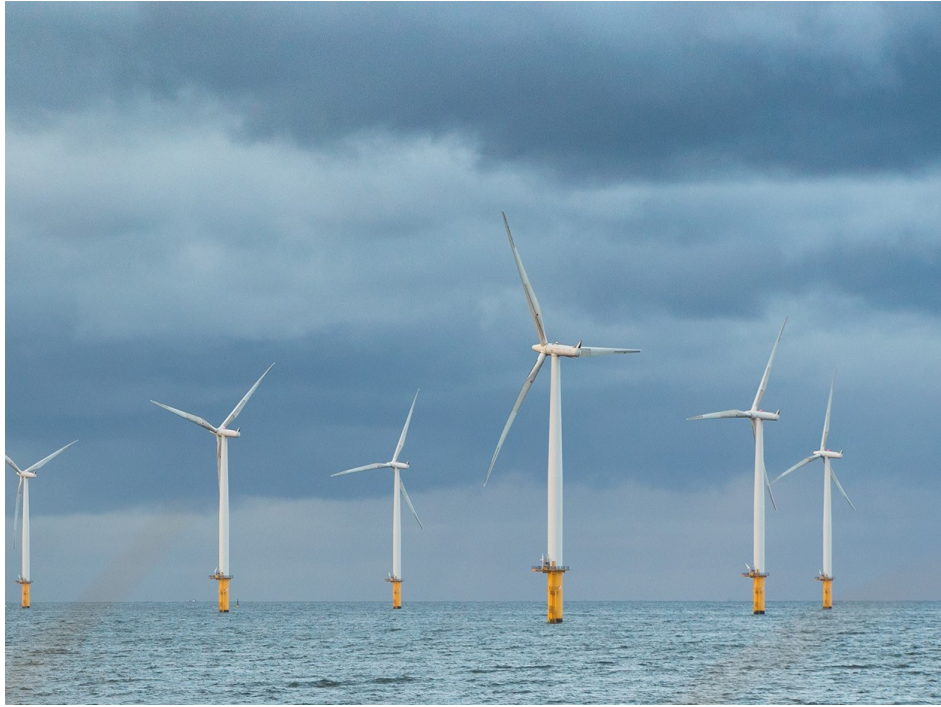
Figure 6.1: View of the turbines supported by monopiles of the Teesside wind farm, copyright EDF Renewables UK.
